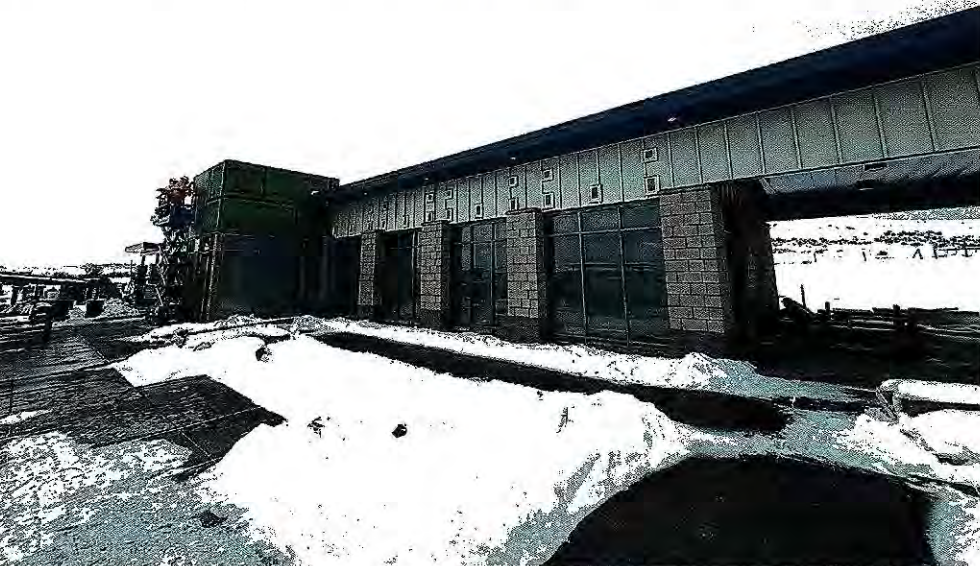
Westbound Hardin Rest Area – Exterior Finishes (Dick Anderson Construction/Tyler Hansen)
