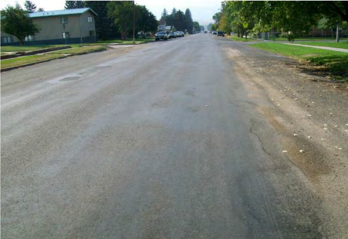
Milwaukee Ave at Clagett St PASER-7
