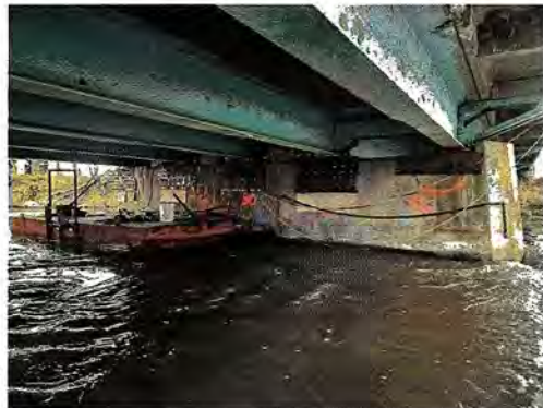
Pictured above: Bridge repairs near completion on Friday, with some beam sets finished and some waiting for epoxy to dry before finishing.
