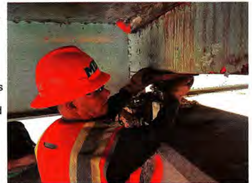
Pictured above: Dave Crumley setting up a bridge jack.
