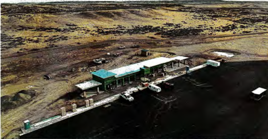
Westbound Hardin Rest Area site. (Dick Anderson Construction/Tyler Hansen)
